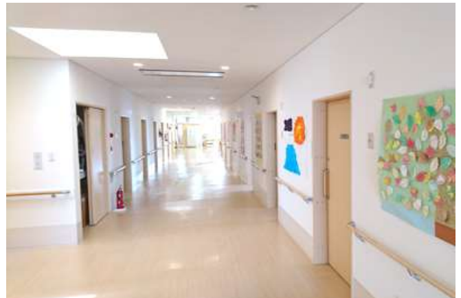
廊下幅は2.7m
